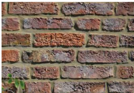
Frampton brick (the traditional brick of the parish)
