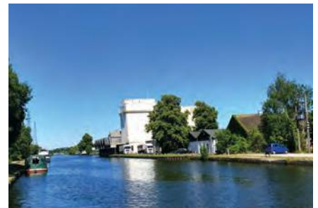
The buildings of the former Cadbury site, now Frampton Industrial Estate
