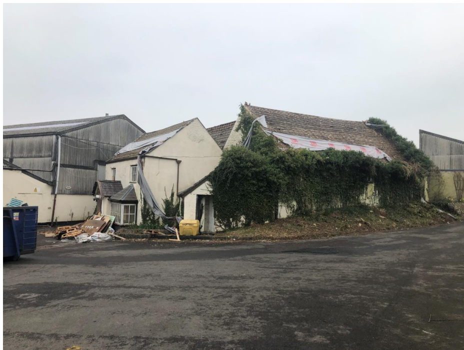
FIGURE 3: PHOTO OF EXISTING BUILDINGS
