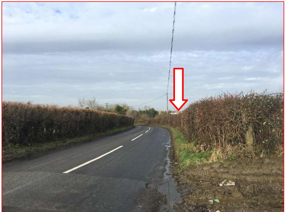
Plate 5 View looking north-west along Hillesley Road. Note that the subject site (arrowed), located to the north-east of the hedgerow (right of picture) is only glimpsed in this view.
