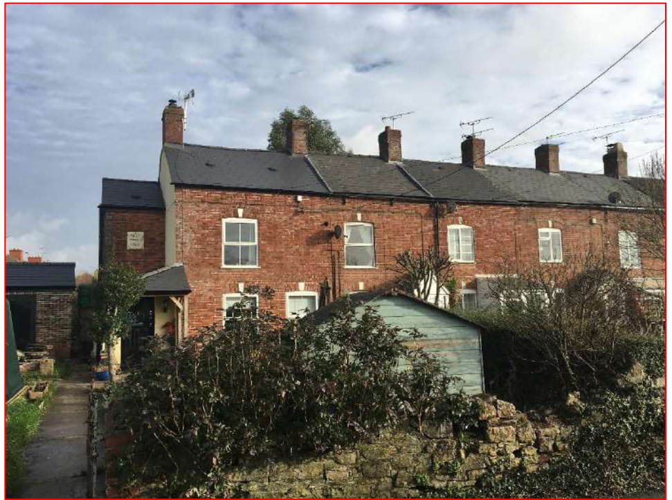
Plate 6 View of late 19 th century terrace group located on east side of Crow Meadow (Rose Terrace). Note that this group is located within the Kingswood Conservation Area, with the southernmost part of this group adjoining the subject site.
