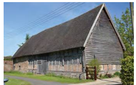
Grade 2* listed barn, part Frampton brick with square interwoven wattle panels Photograph by Joy Greenwood
