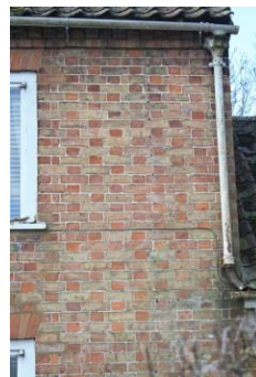
Old brickwork, Lower Wick
