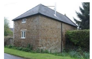
Stable conversion, Lower Wick
