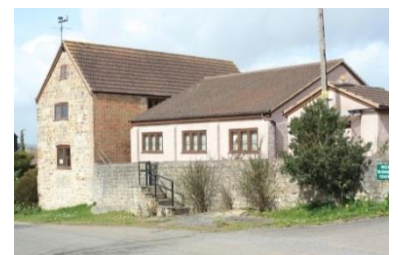
Business units in redundant farm buildings, Upper Wick
