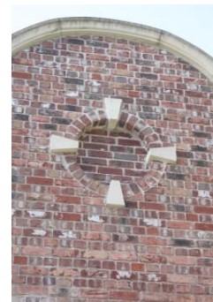
Recycled brickwork detail on a new garage extension, The Myrtles, Chapel Hill
