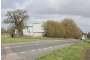
Approaching Newport from the south showing the large industrial units
