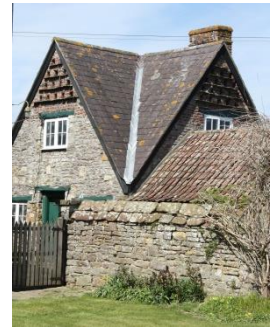
Oakleaze Pump house, Swanley
