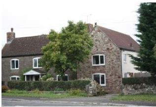
Stone building to the west of the A38 showing a more recent extension to the right Woodford
