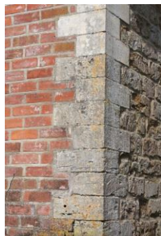
Brickwork & stone used together Lower Wick
