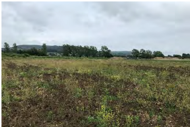
Reworked ground in northern area.
