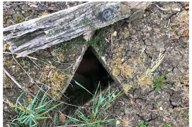
Drainage outlets under concrete cover in northeast.
