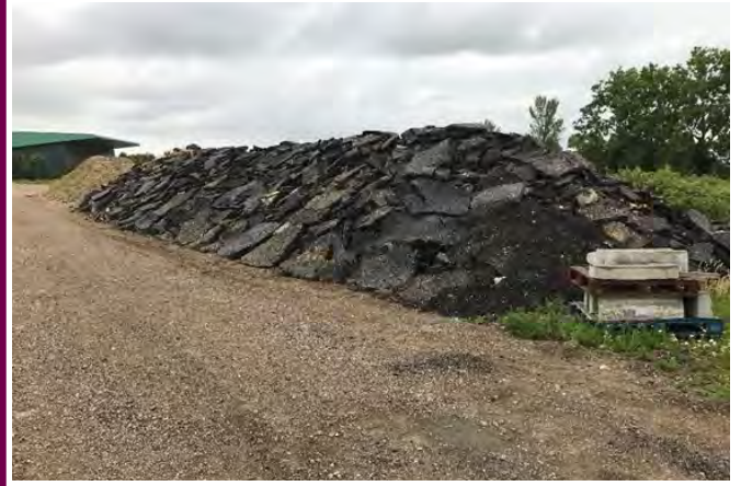
Tarmacadam and soil stockpiles .
