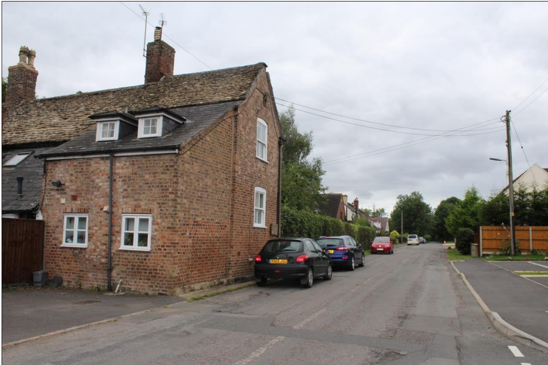
Figure 12 View of LB2 to LB4 from Dursley Road looking south-west towards the Site (specifically Parcel D)
