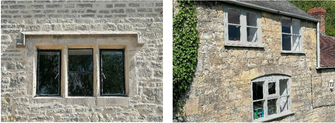
Plate 30 (left) Example of a Stone Mullion window and plate 31 (right) Example of a casement timber window
