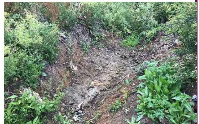
Drainage ditch on northwestern boundary.
