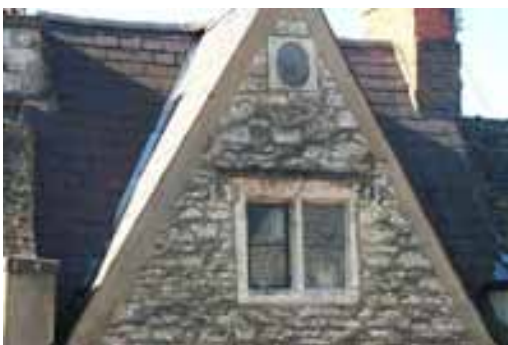
Above: A steeply pitched gable demonstrating key characteristics local to Stroud; stone mullion window, drip mould and small oval window inserted into the apex of the gable
