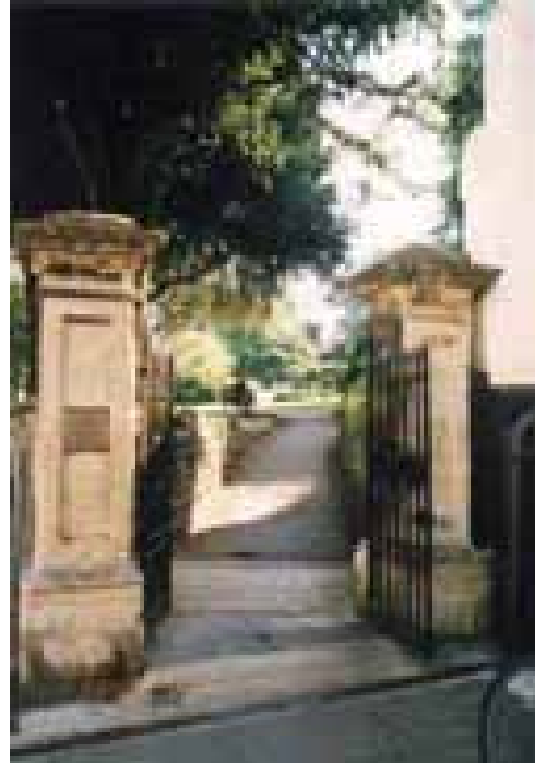
Above: The impressive stone gate piers and iron gates, which lead into Bank Gardens
