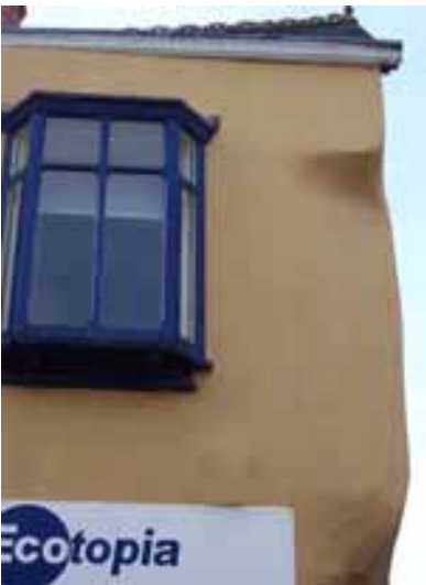
Left: Timber framed jetty on the High Street
