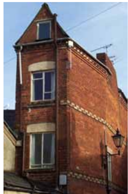
Right: An interesting use of brick banding, adding further interest and variety to this already quirky 19 th century building
