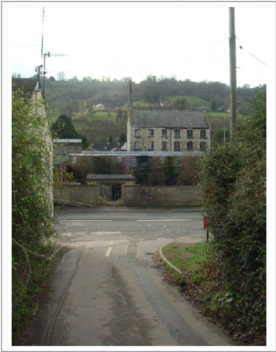
below: Whilst this mill complex is characteristic of the lack of positive canal frontage or canal orientation in the conservation area, the image it presents to the tow path is not a good setting for the historic buildings on the site. Large expanses of tarmac, modern industrial sheds, a lack of enclosure and wire fencing all leave plenty of scope for enhancement
