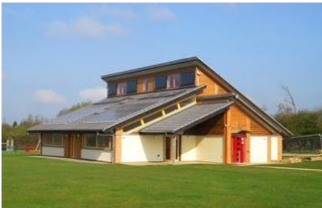
[Solar Panels on community hall at OHMG]
