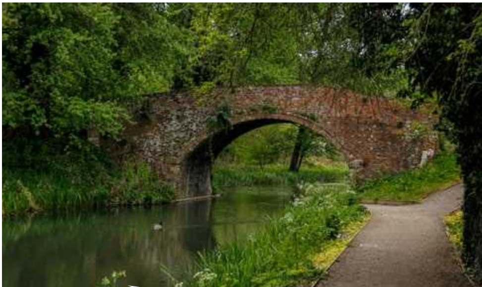
Image 30: Bridge over Severn Thames Canal
