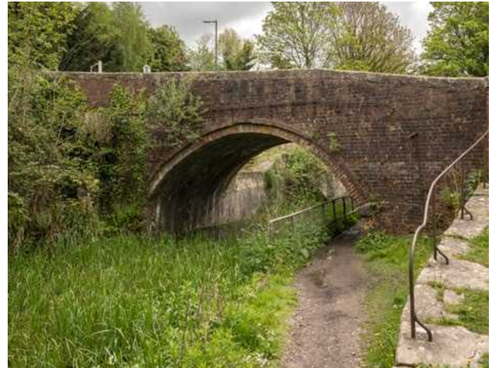
Image 51: Bridge over the Severn Thames Canal
