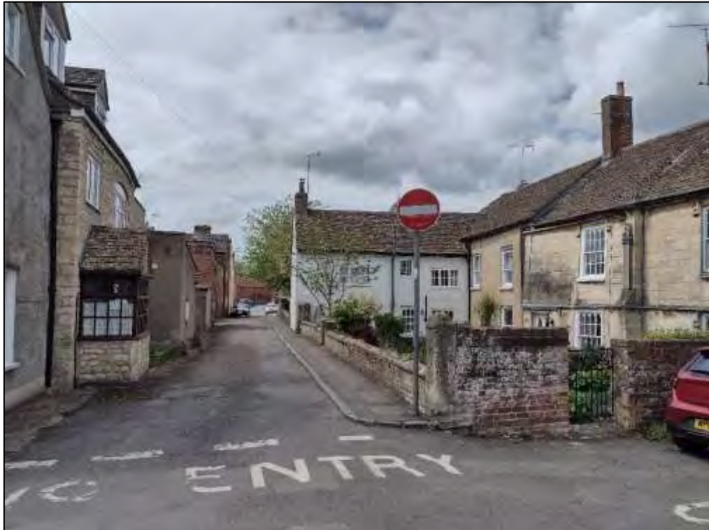
Photo 14. Historic core of Kingswood Conservation Area north-west looking towards Site
