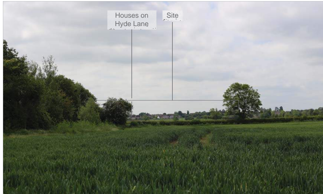
Viewpoint 9. Looking south from Footpath EWH12 to the south of Moreton Valence (approximately 700m from the site)
