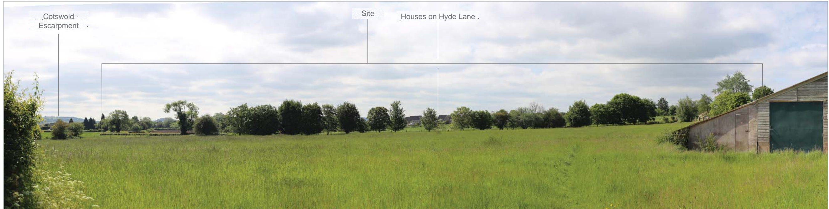
Viewpoint 11. Looking south from Footpath EWH12 in the field to the north of the site (approximately 140m from the site)
