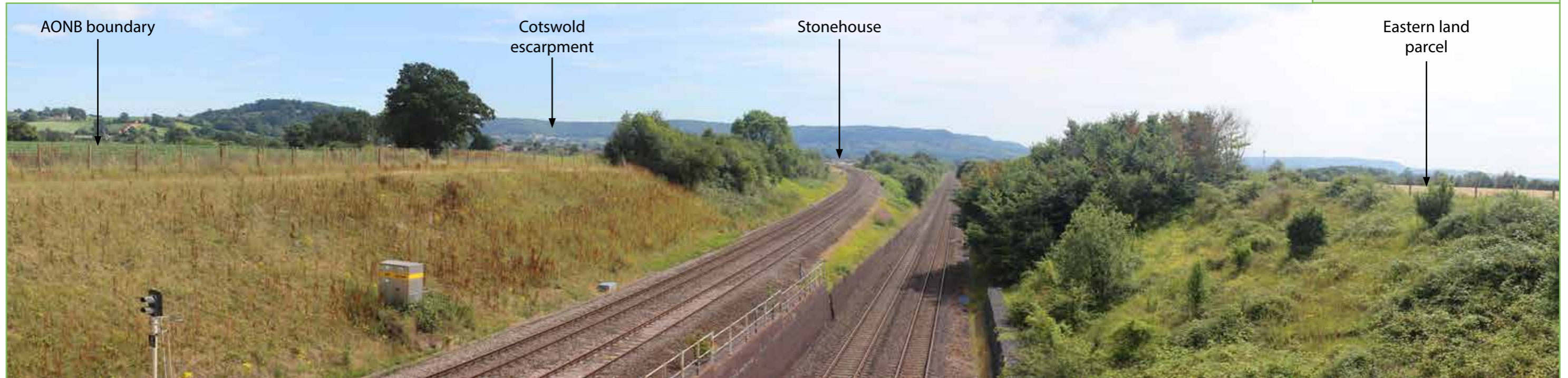
View looking south from Black Bridge
