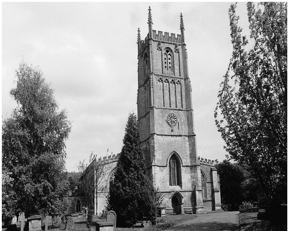
Photo 15 – St Mary the Virgin, Culverhay. The six stage tower, with the two upper stages dating from around 1371, is described in Pevsners "The Buildings of England" as "one of the most splendid perpendicular towers in the county".
