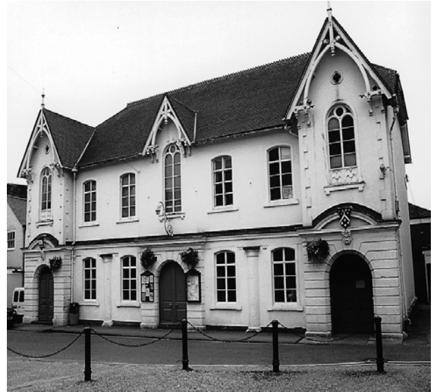
Photo 11 – Town Hall. This C17 building underwent major reconstruction in 1872. It was formerly an open sided market hall beneath an upper floor town hall. The open sides have now been fully enclosed, but the originally freestanding columns are still clearly visible.
