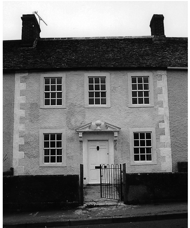
Photo 13 – No. 9 The Chipping – the central house in an informal terrace of three, dating from the early C18. The render has recently been limewashed, the traditional finish for rendered buildings. This group is vital to the visual enclosure of The Chipping
