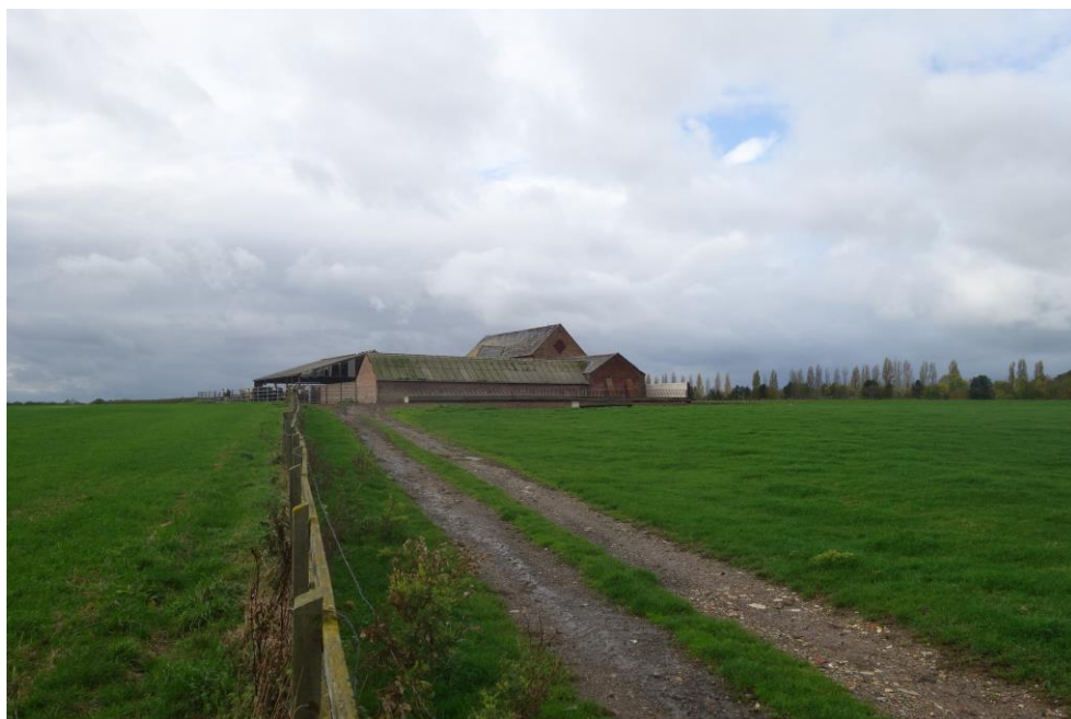
Plate 27: View looking S along trackway from Daniel's Brook towards Field Buildings
