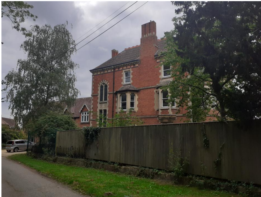
Plate 29: Oblique view W along Church Lane showing SE facing elevation of house
