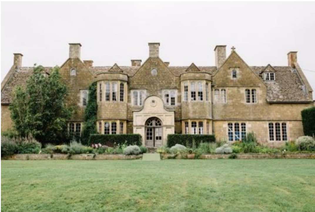
Plate 19: View looking W across lawned garden towards the front of Hilles House
