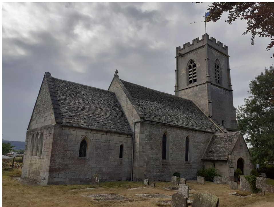
Plate 9: View SW towards St Margaret's Church showing N porch
