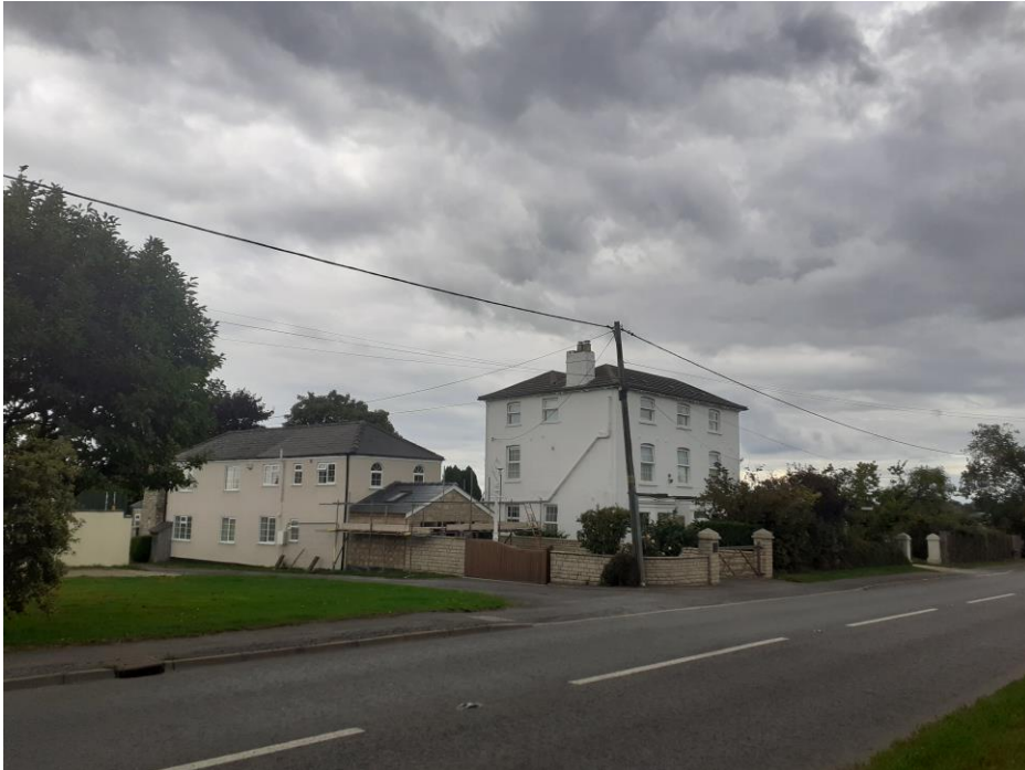
Plate 32: View looking NW from Stroud Road towards Brook Farmhouse
