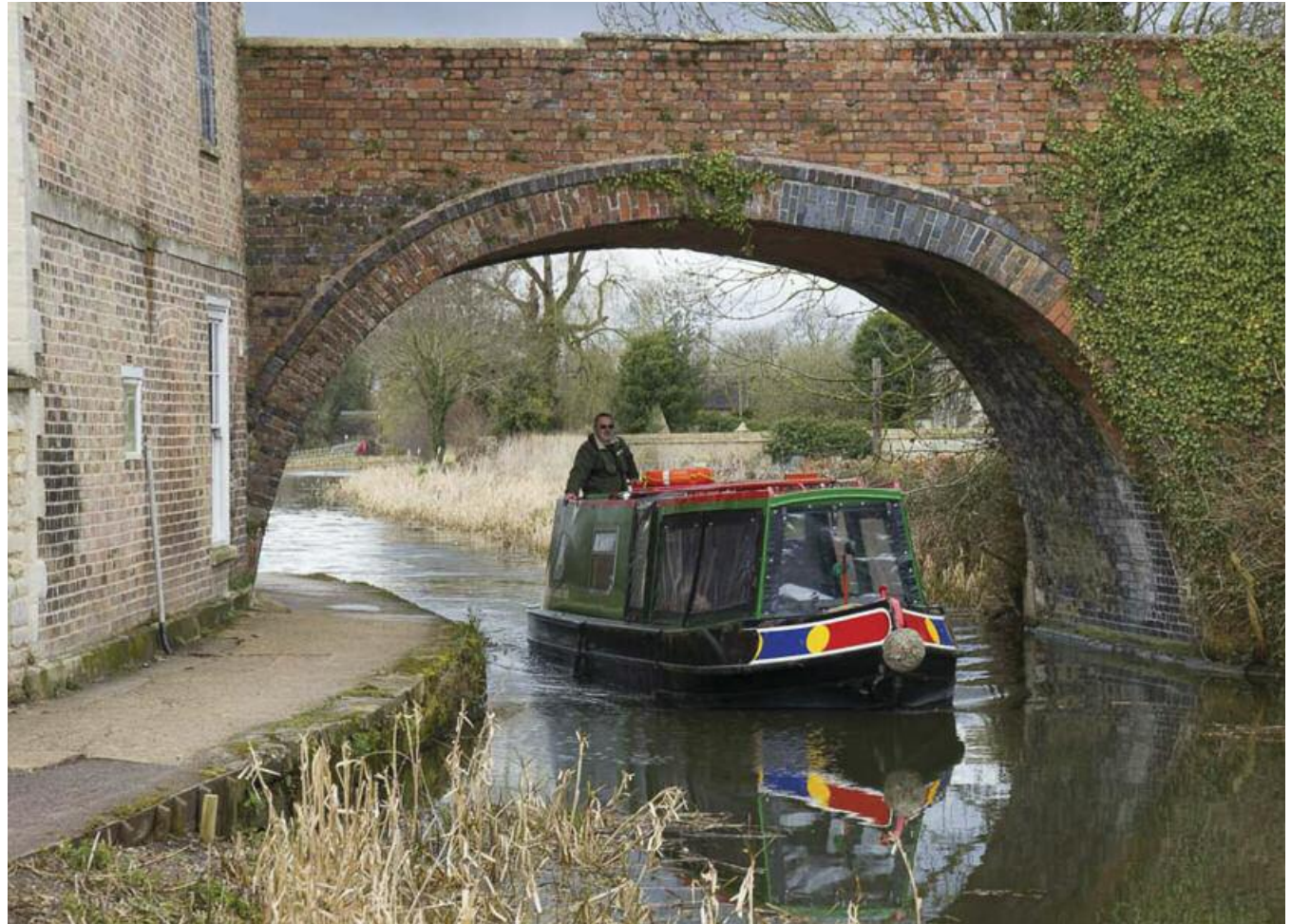
Nutshell Bridge on the Stroudwater canal
