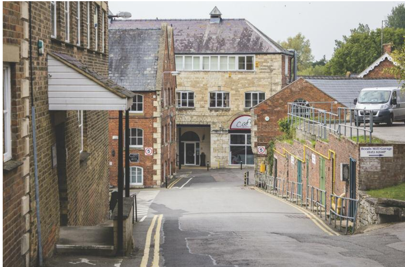
Units at Bonds Mill Estate
